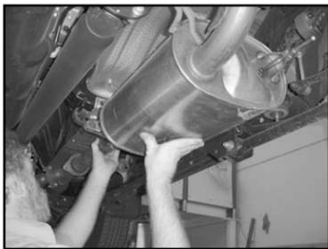
8. Insert the JBA intermediate pipe (A) hangers into the (2) rubber isolators then bolt the intermediate pipe to the factory catalytic converter assembly using the factory hardware.
